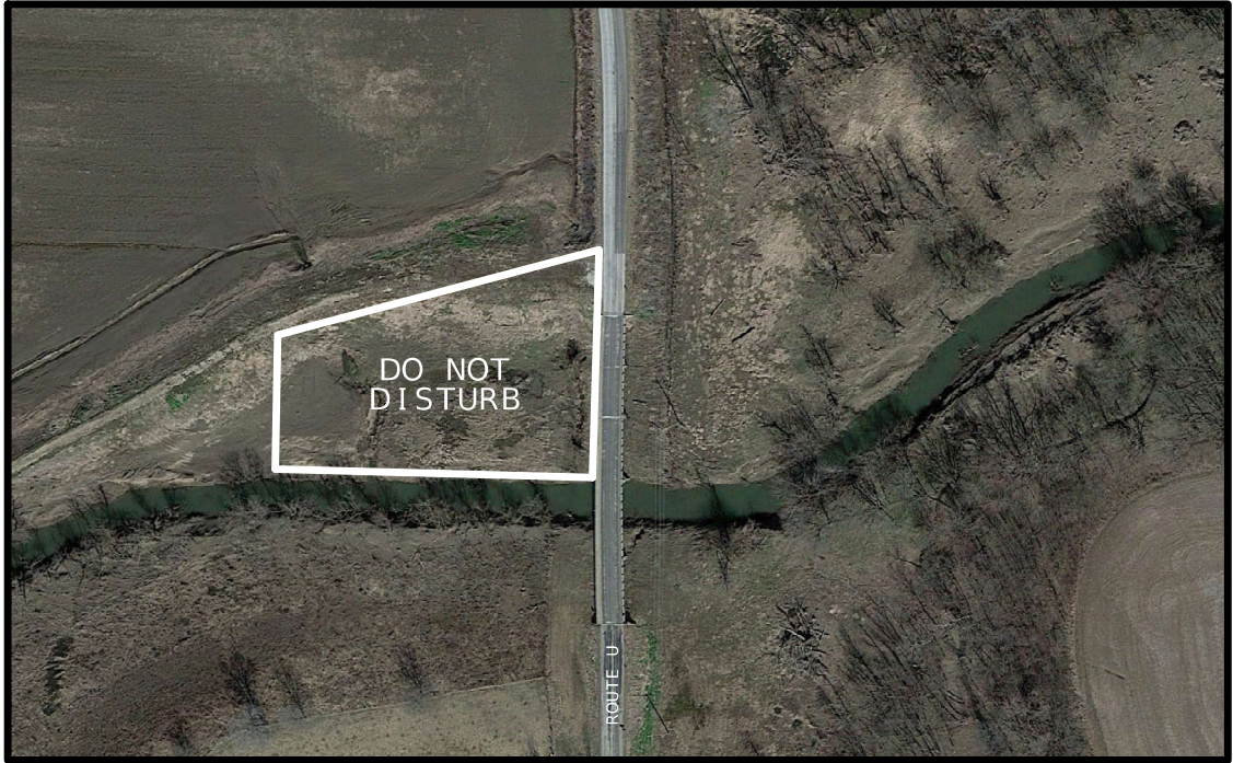
BRIDGE #N0983 ROUTE U OVER PETITE SALINE CREEK
