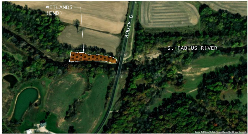
BRIDGE B0198 MARION COUNTY ROUTE D
