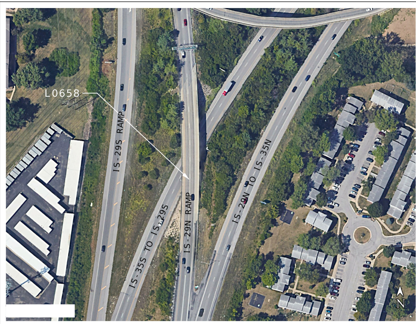
L0658: I-295 NB RAMP TO I-295 NB AT I-35 INTERCHANGE
