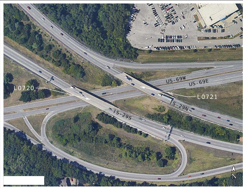
L0720: I-295 SB OVER US-69 L0721: I-295 NB OVER US-69
