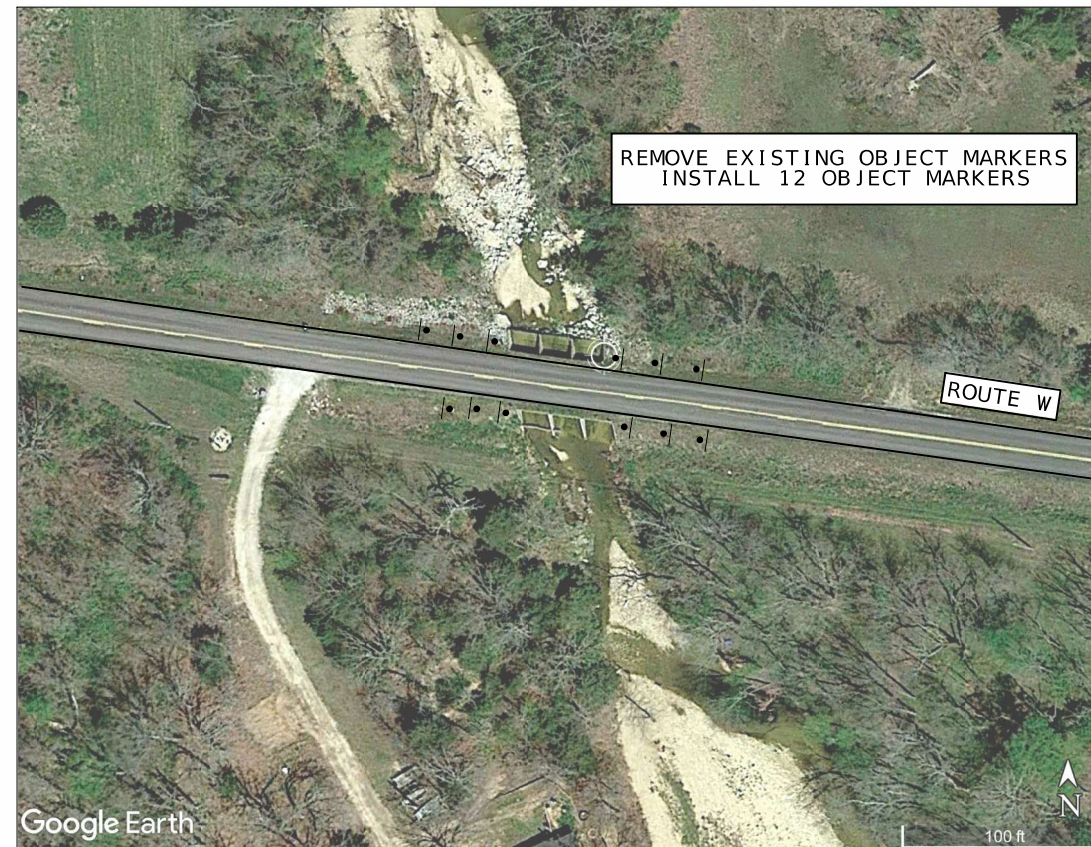
ROUTE W - CULVERT N0979 - LOG MILE 2.349
