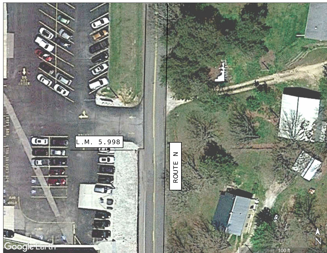
ROUTE N - BEGIN WIDENING - LOG MILE 5.998
