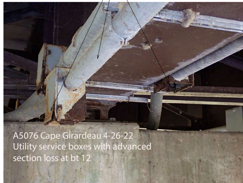
CONDUIT REPAIRS AT EXPANSION JOINTS (Bents No. 1, 4, 5, 9, 12 and 15)
