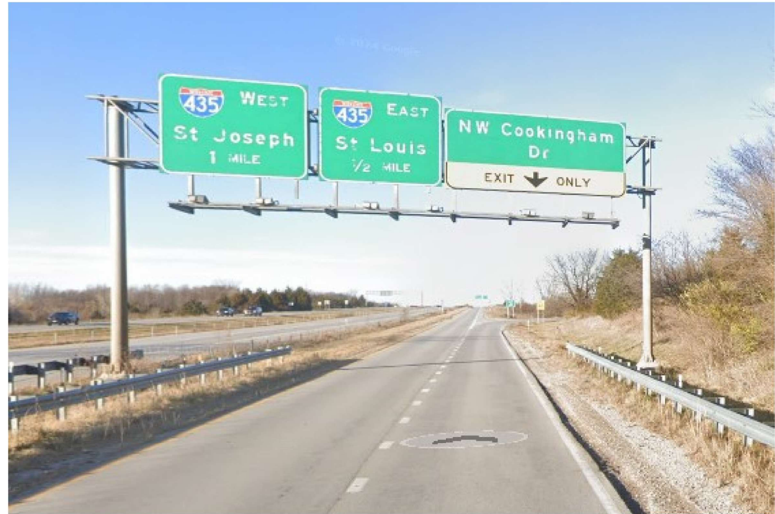
REMOVAL OF IMPROVEMENTS CATWALK/LIGHTING
