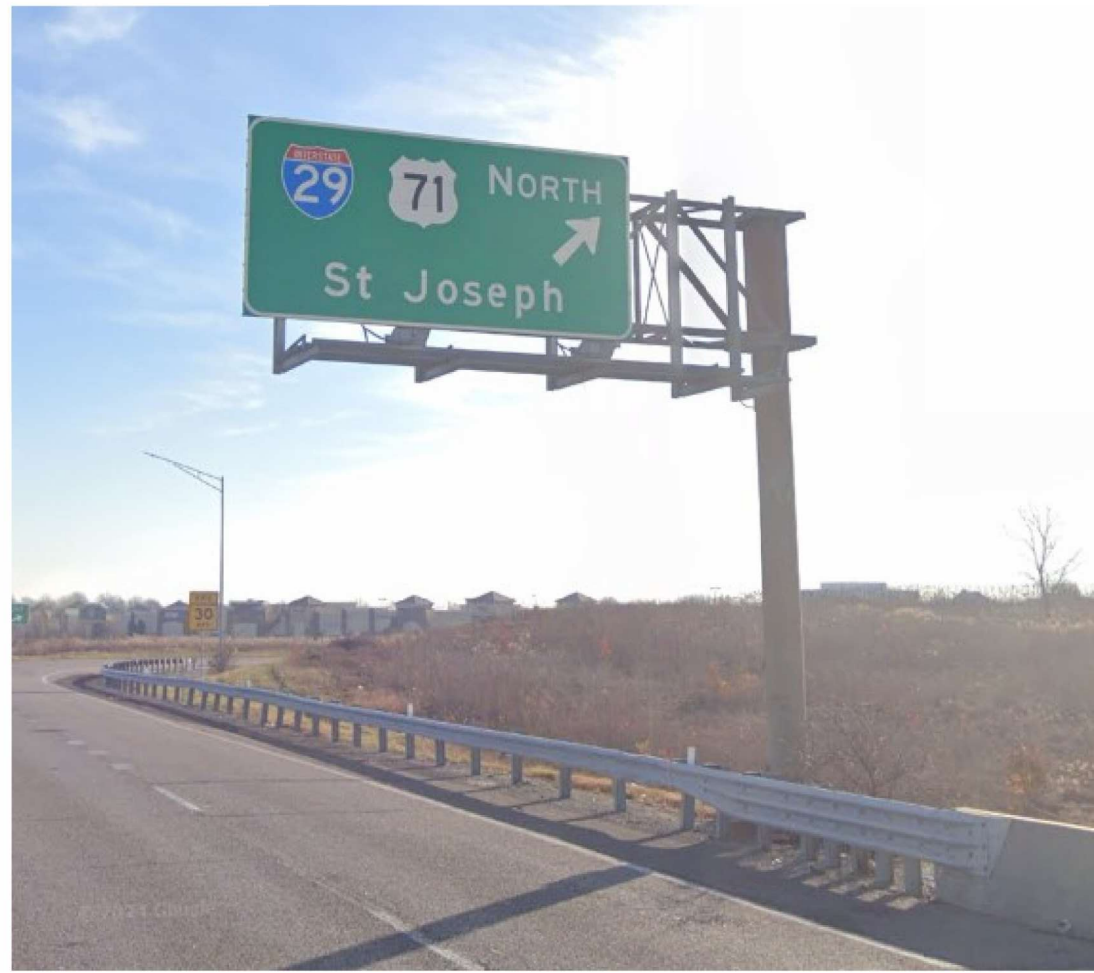
REMOVAL OF IMPROVEMENTS CATWALK / LIGHTING
