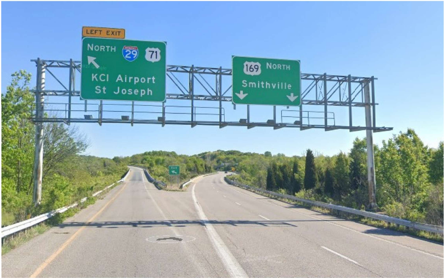
REMOVAL OF IMPROVEMENTS CATWALK/LIGHTING
