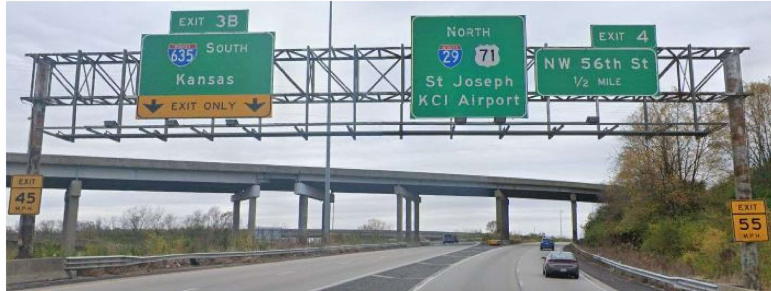
REMOVAL OF IMPROVEMENTS CATWALK/LIGHTING
