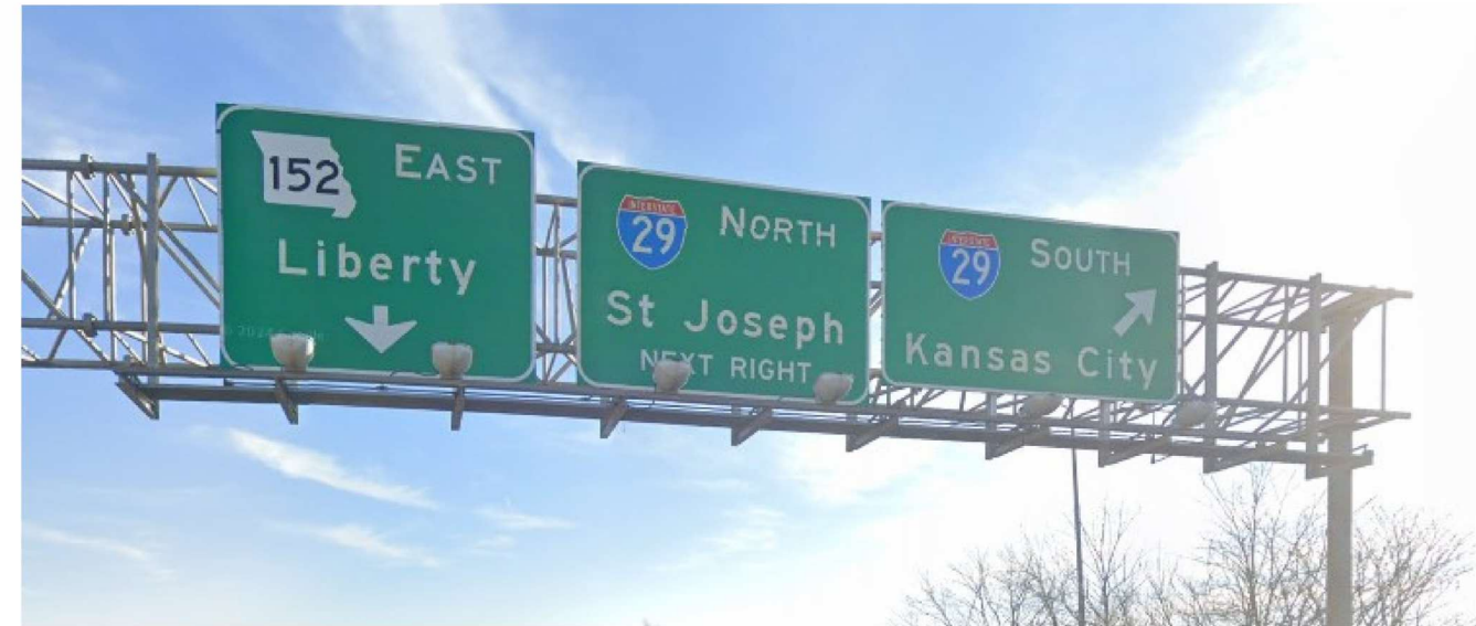
REMOVAL OF IMPROVEMENTS CATWALK / LIGHTING
