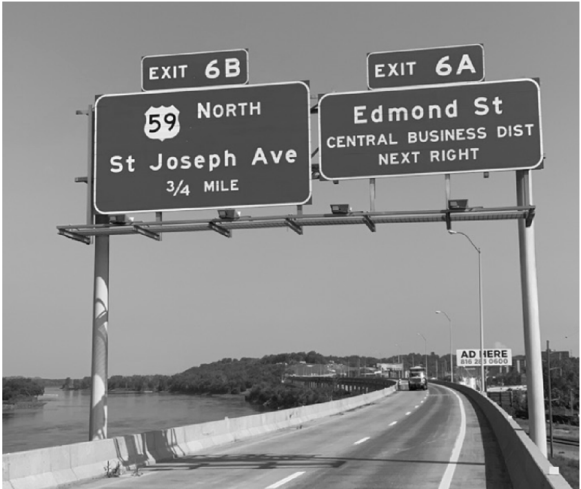
REMOVAL OF IMPROVEMENTS
