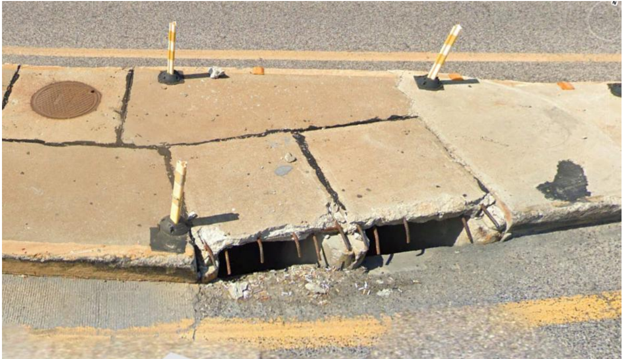
EB MO 30 Left Turn Lane to NB I-270 Ramp
