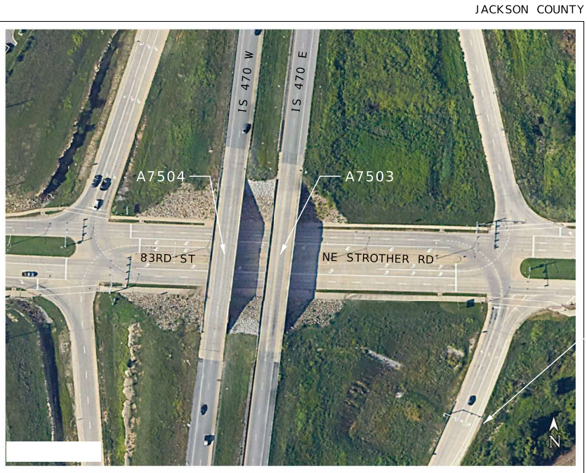
A7503: IS 470 E OVER CST NE STROTHER RD A7504: IS 470 W OVER CST NE STROTHER RD
