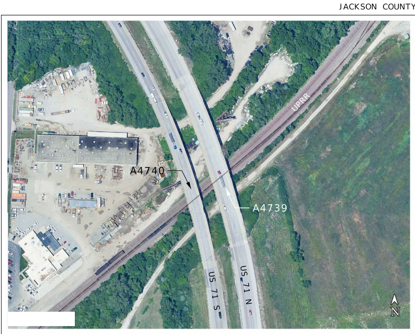
A4739: US 71 N OVER UPRR A4740: US 71 S OVER UPRR
