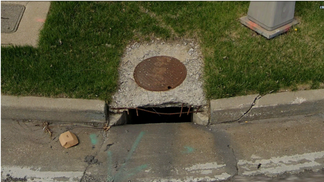
Northwest quadrant of Clarkson Road with Manchester Road in SB Right Turn Lane
